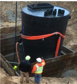
The Weholite wet well was delivered to the project requiring no internal plumbing or cast-in-place base work. The wet well vessel was ready to be set, connected, and backfilled immediately upon delivery.
